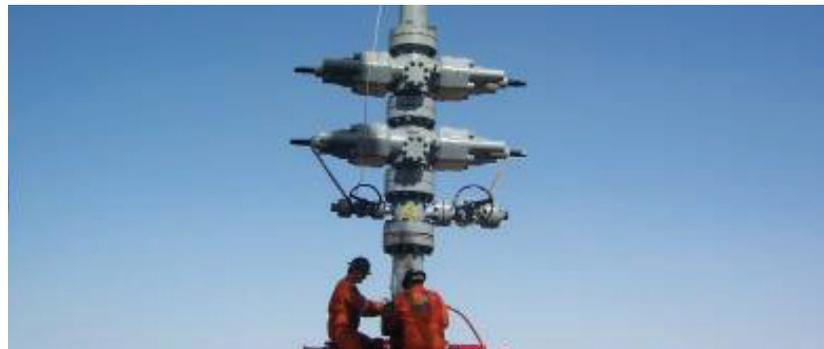
The rig was skidded using two two traveling blocks and a deadman system strung together with 1 1/8" drill line. After removing the annular BOP the tubing was again jet cut approximately 6" above the rig's double BOP to allow for the capping stack to be spun on over the flow.
